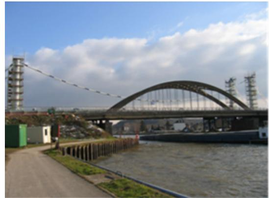
Fig. 6 - First cable installed / Premier câble en place
