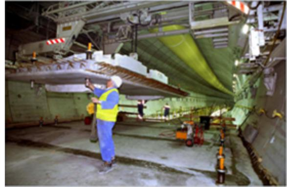
*Once placed, precast elements are connected by cast in situ joints every 2.67 metres, and completed by cast in situ edges in order to match perfectly the tunnel lining.*
