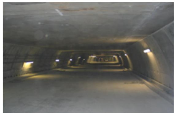
*As it is the case with the lower slab, transverse joints are left every 200 metres during construction in order to allow early deformations, mainly shrinkage.*
