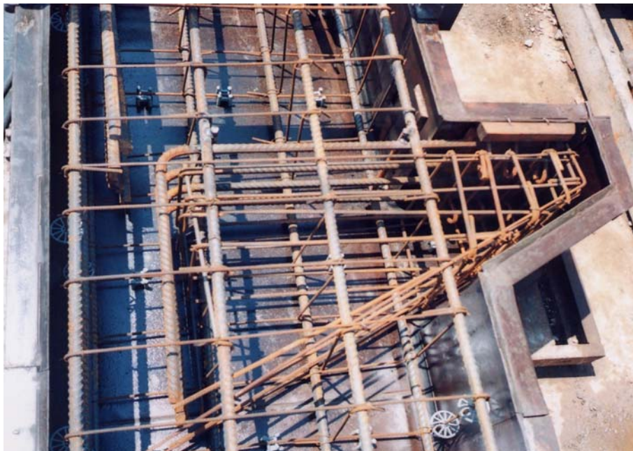
Fig. 9-18: Reinforcement arrangement for corbel
