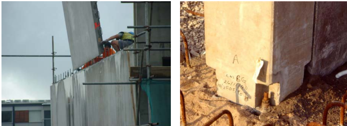
Fig. 1-2: Grouted dowels (left) and bolted steel plates are just two ways of making mechanical connections
