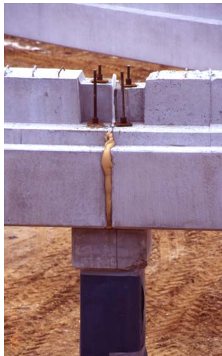
Fig. 9-27: Construction of beam-column head connection
