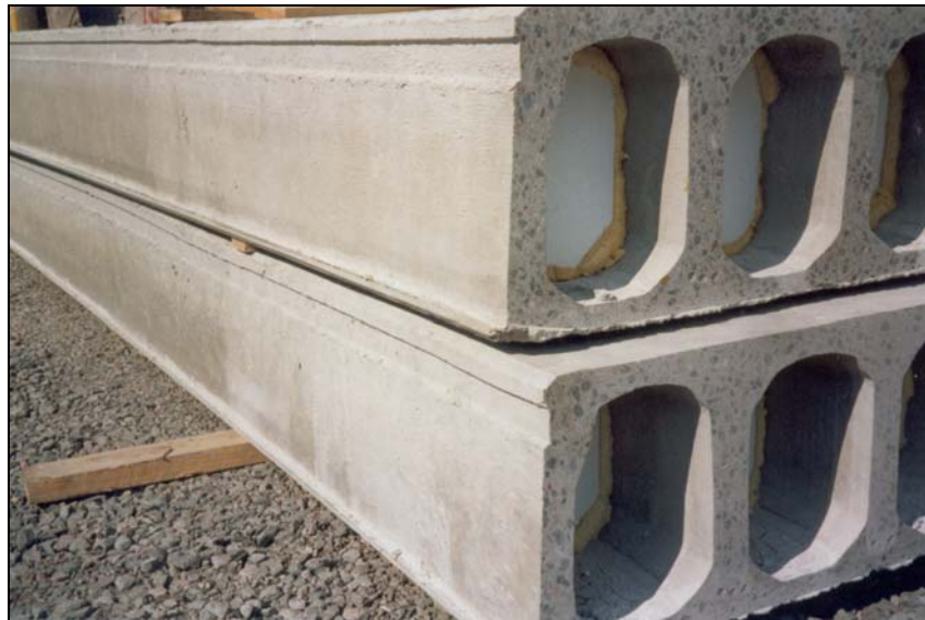
Fig. 8-62: Edge surface at longitudinal joint face. Photo: authors
