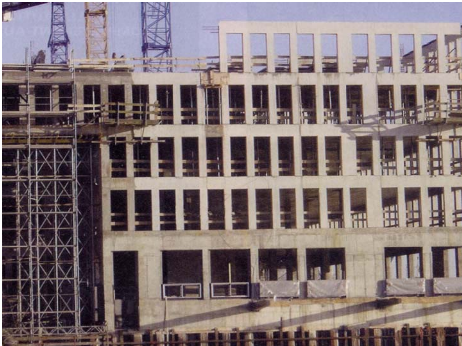
Fig. 9-1: Moment resisting perimeter frame (Courtesy BFT Journal)
