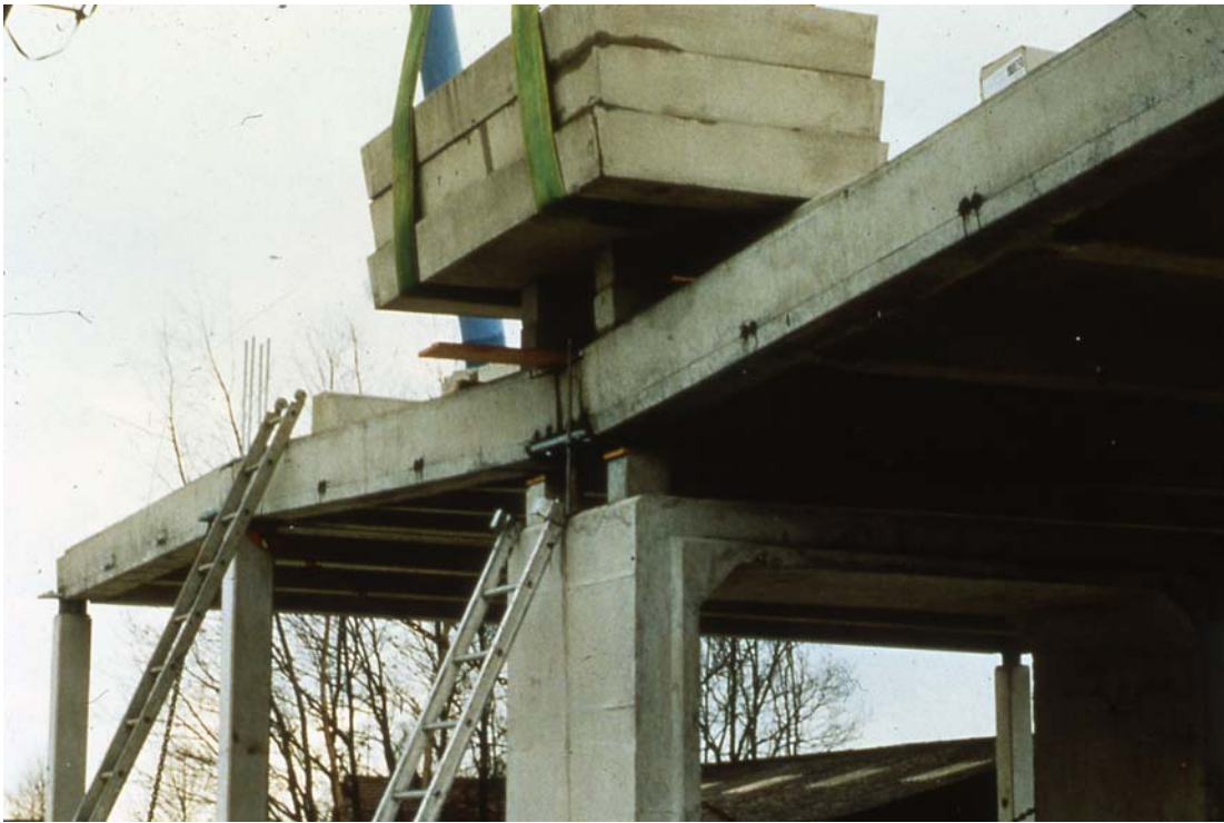
Fig. 5-18: Test of demountable precast concrete system 'Matrixbouw', The Netherlands for alternative load path and redundancy
