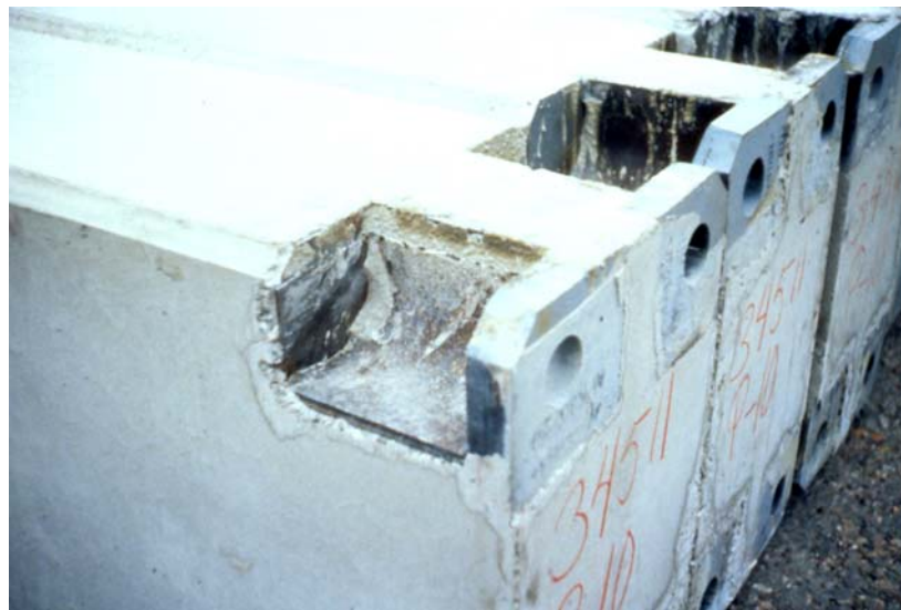
Fig. 9-34: Column splice shoes cast into the bottom ends of a column (or wall)
