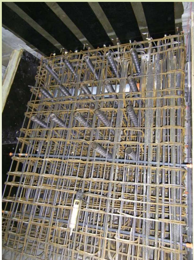
Ferrailage massif ancrage
