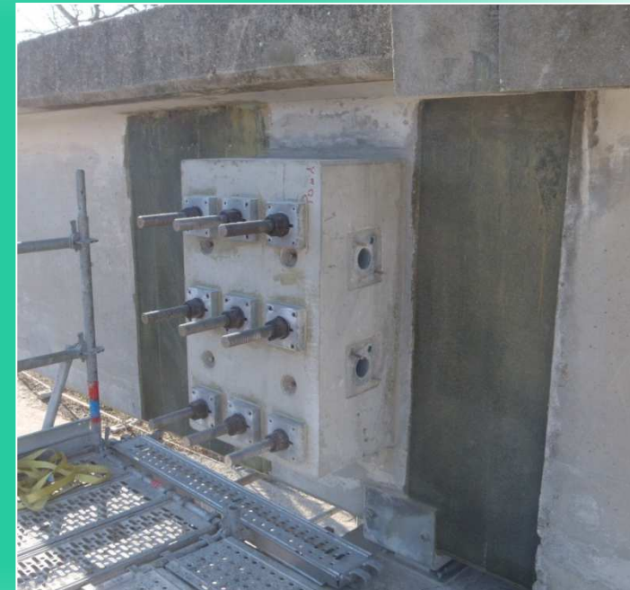
Blochet + renforcement composite
