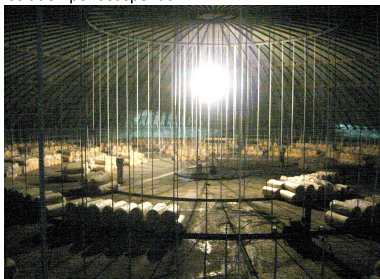
Isolation pont suspendu
