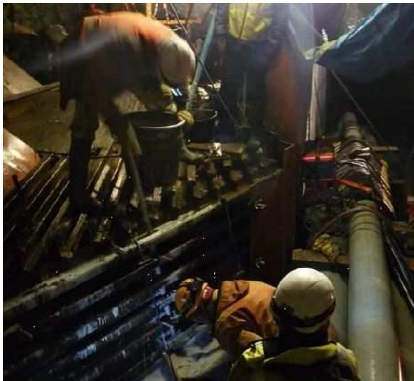
Figure 11: Casting of UHPFRC between railways during the winter of 2012.
