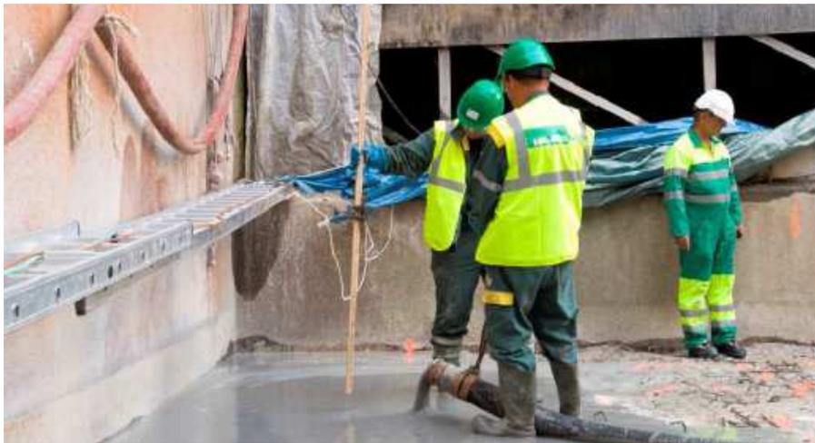
Figure 4: UHPFRC casted with the pump on the Caderousse Dam.
