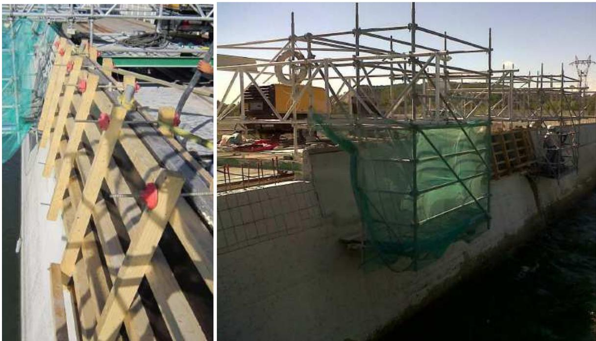
Figure 7: UHPFRC casting (with injection hole) and 2 scaffolds on Beaucaire Dam.
