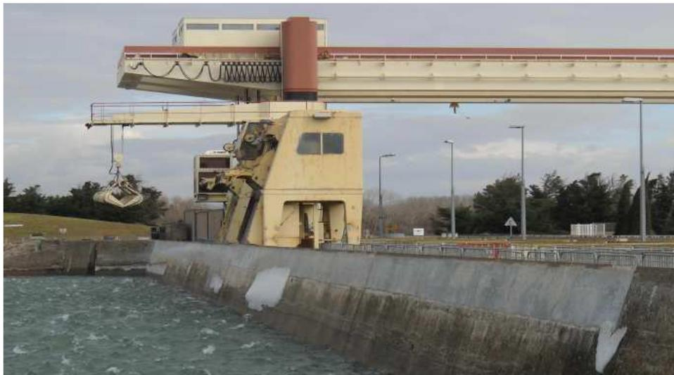
Figure 5: Caderousse Dam's screen rakes after completion of UHPFRC repairs (light grey portion).
