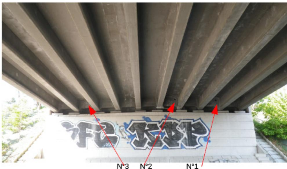
Figure 5: Cores drilled from OA6 bridge in the cross-beam above abutment
