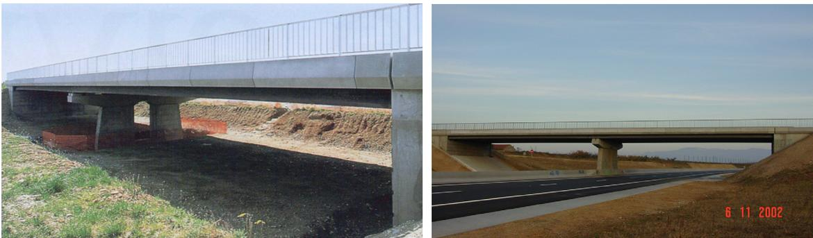
Figure 1: UHPFRC bridges under completion at Bourg-lès-Valence
