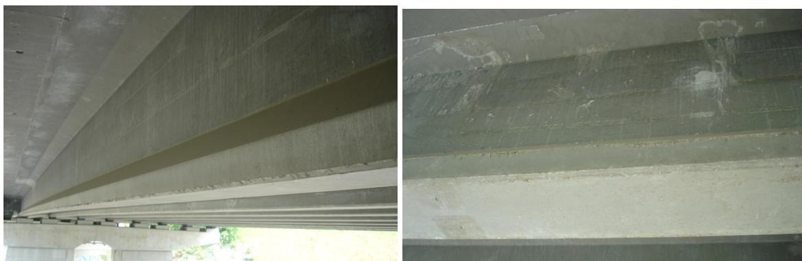
Figure 4: Pi-shaped UHPFRC beams facings
