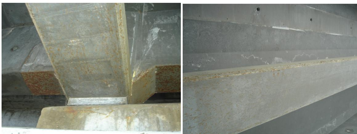
Figure 3: a) Effect of water stagnations over abutments (left)
