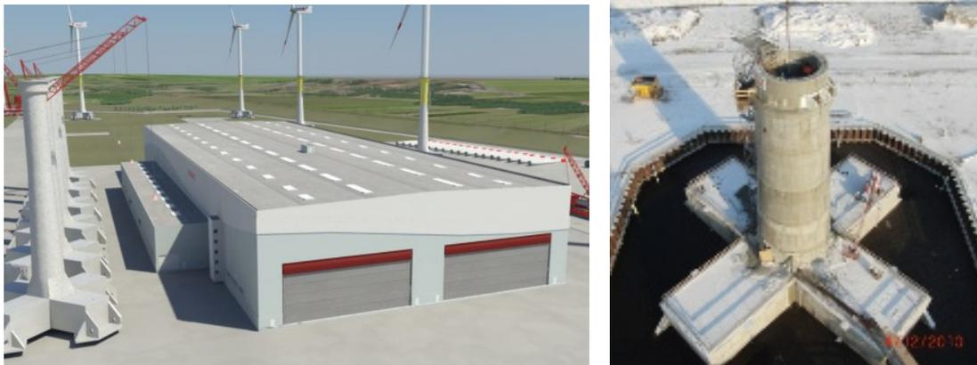
Figure 1: STRABAG Terminal in Cuxhaven (left) and full-scale model of STRABAG Gravity Base Foundation (right) [4]
