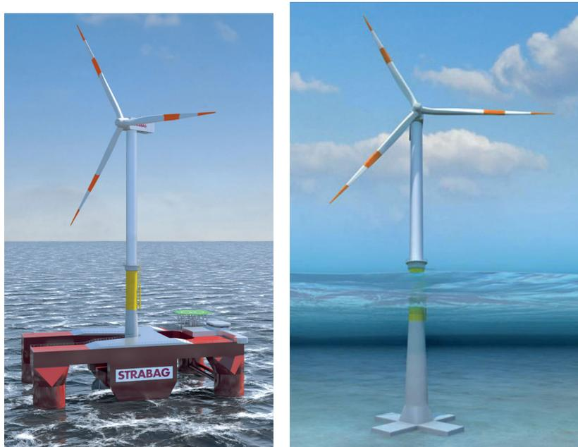
Figure 2: STRABAG Carrier (left) and STRABAG Gravity Base Foundation with steel tower installed at operating site (right) [5]
