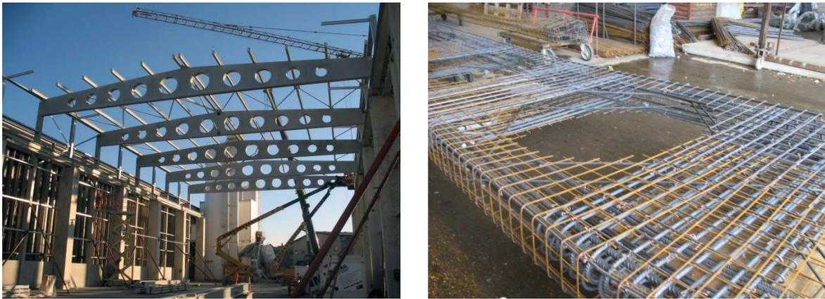
Figure 1: Cellular beams and corresponding passive reinforcement
