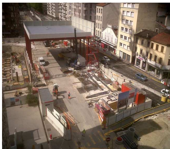
Installation du chantier Incity
