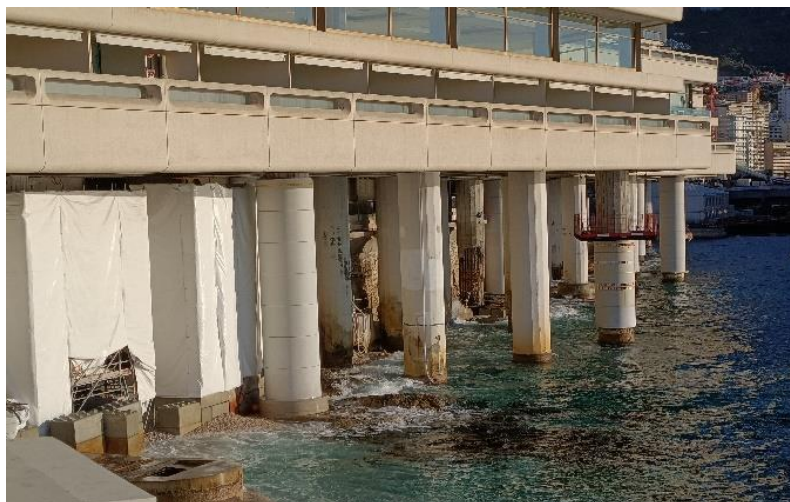
Reinforcement of the Spelugues piers © J.Resplendino
