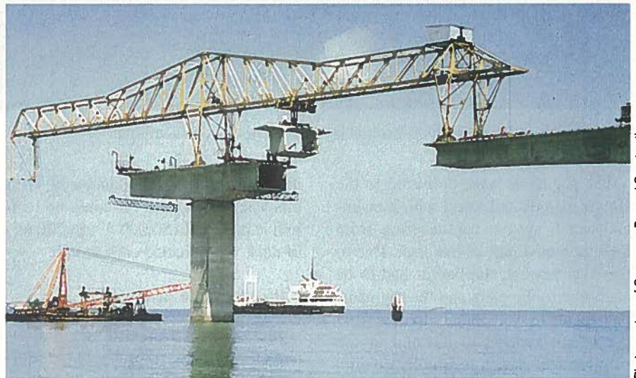
Fig. 8. The Oleron Bridge connects Oleron island to mainland France.
