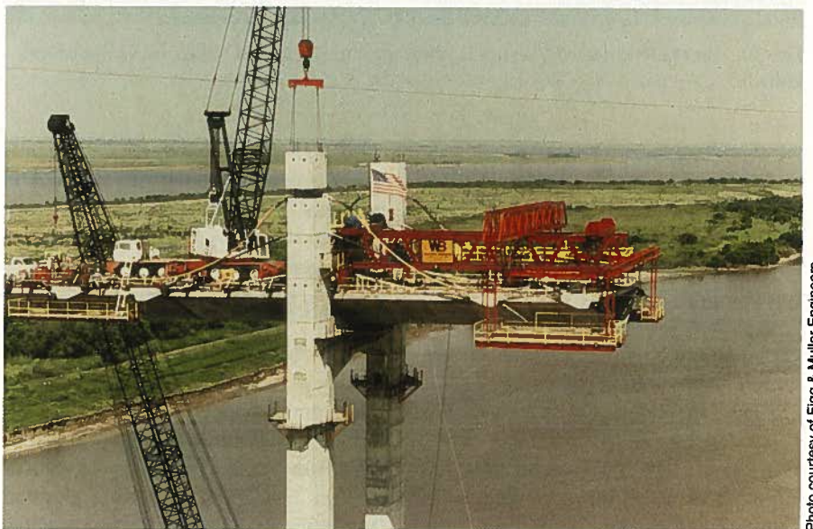
Fig. 20. Pictured is the Neches River Bridge precast concrete pylon in Texas.
