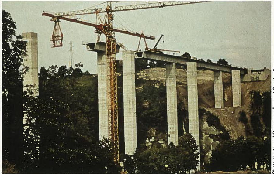
Fig. 12. Shown is the Alpine Motorways viaduct in France.
