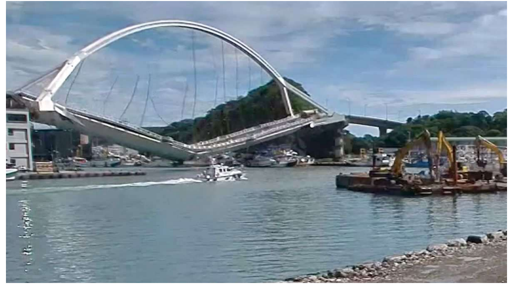
2019 : nanfang'ao bridge collapse : ( Corrosion )
